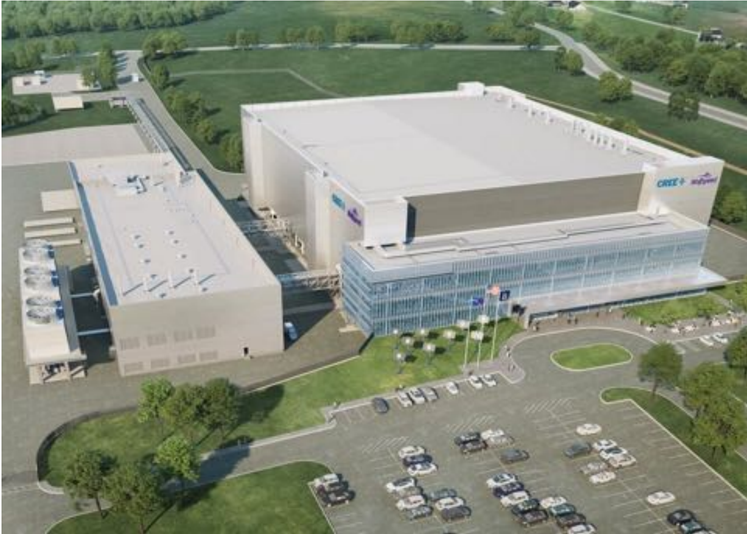
Cree - $1B Silicon carbide fab under construction
